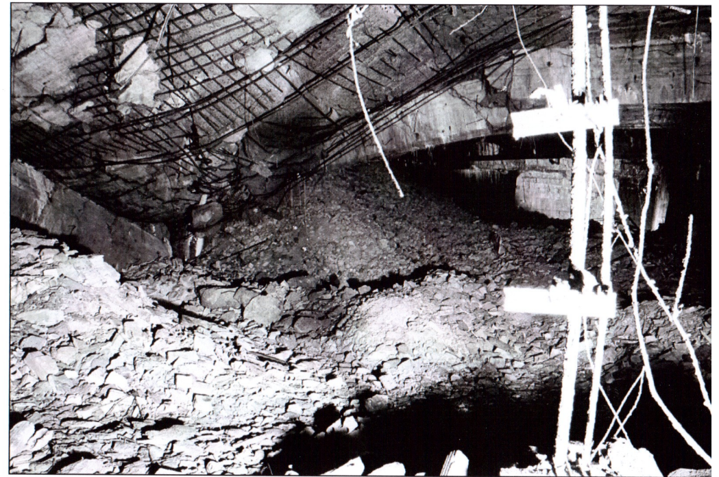
Left: He's not drunk and not on a ship, the stairway is slanting at an angle. Top: The dense reinforcement in the ceiling holds the concrete together. Bottom: Piles of rubble from the shattered interior constructions, which were built of bricks and mortar
