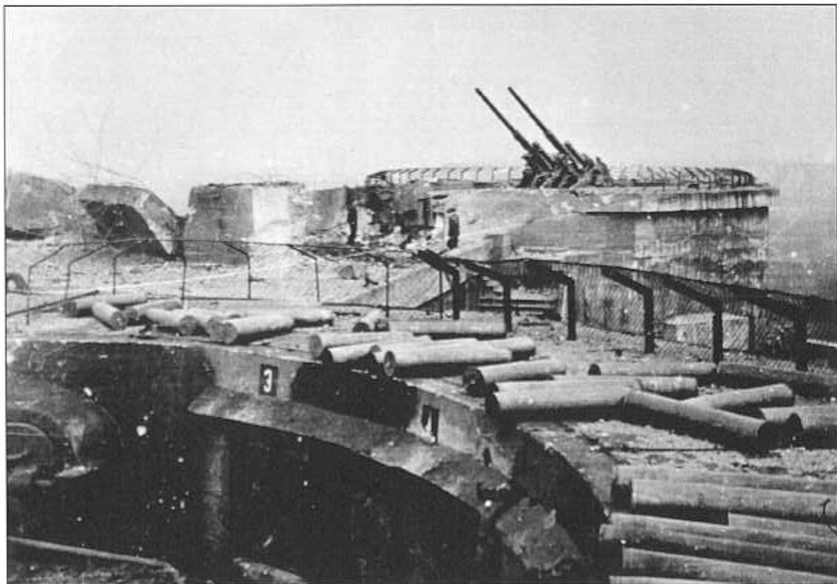
The ammunition chamber of Gun "Cäsar" of the G-tower Friedrichshain received a direct hit on February 3 rd 1945, causing the explosion of 400 calibre 128 mm shells. Nine Luftwaffenhelfer from Berlin died. More serious were the two direct hits on March 18 th 1945 on tower A and D (bottom) of the Humboldthain G-tower. The damaged 128 mm guns could be repaired and used again. It is lucky the direct hits didn't trigger the 128 mm grenades stored in the ammunition niches, otherwise the whole Flak tower wouldn't have survived.
