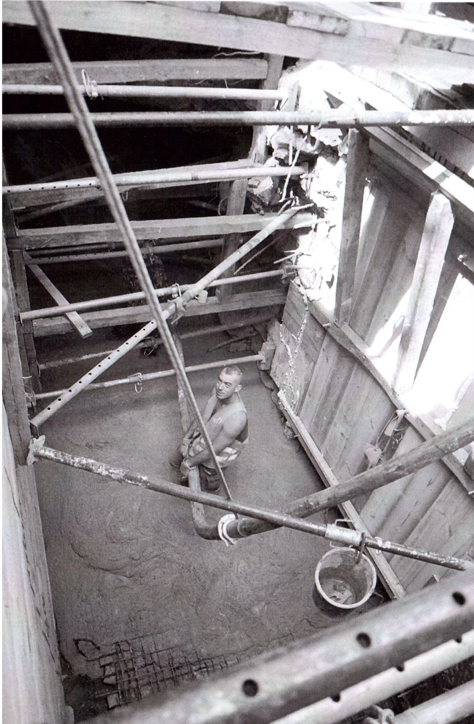
In 2003, the Berlin Underground Worlds' started extensive construction and clearing work to make the G-tower safe for tourists and visitors. Left: concreting the ceiling over the connecting staircase between the 4 th and 5 th floor. Top: Clearing the steps of the connecting staircase. Bottom: The Berlin Underground Worlds' have been running sightseeing tours since April 2004. From October to April the Humboldthain G-tower is closed to allow colonies of protected bats to hibernate the winter sleep undisturbed.
