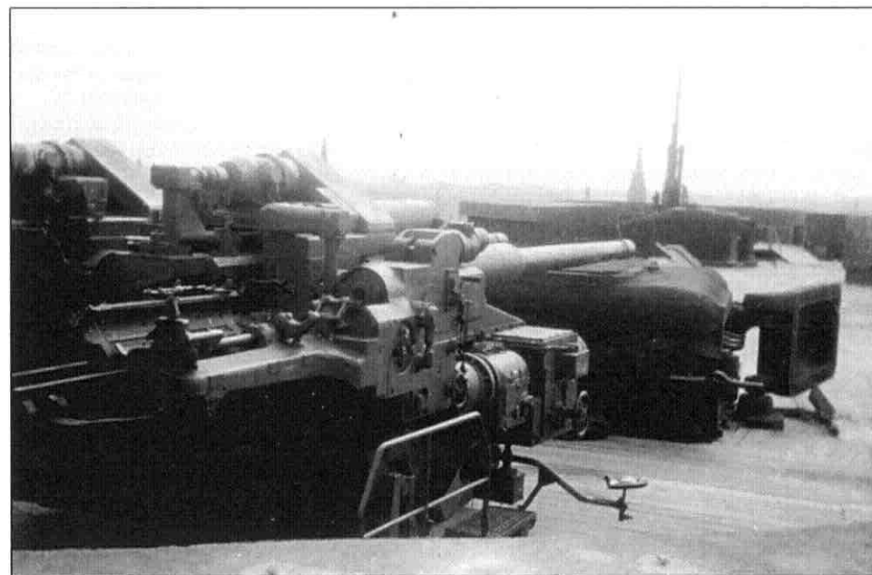
Both the tower crane as well as external cranes were used to lift the heavy 27 tonne AA-guns onto the top of the G-Tower. The guns had to be disassembled first. Top left: Each barrel was transported individually onto the top of the Friedrichshain G-Tower and stored there for a while (top right). Then the first AA-guns were assembled and mounted on their plinths.
