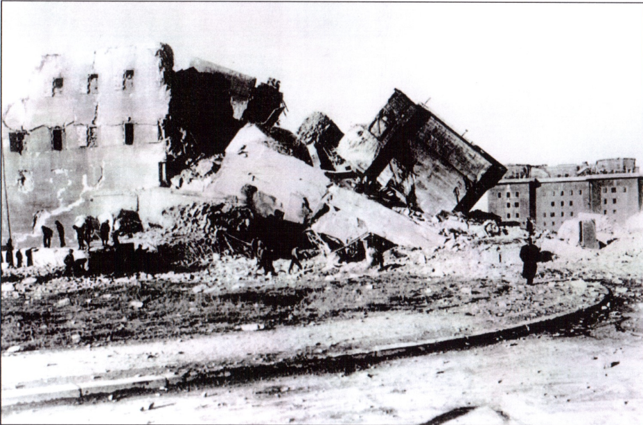
Top: Both southern towers and the outer wall between them collapsed after the third blasting on March 13 th 1948, using 25 tonnes of explosives. Right: Relief workers are covering the Humboldt G-Tower with the debris of 4,000 dwellings or 1.6 million cubic meters of rubble. In 1950 some 1,300 relief workers were employed on the "Rubble Mountain" site. Bottom left: The L-Tower after the blast on December 13 th 1947 which used 16 tonnes of explosives. The upper row of windows and the wall fragment can still be seen today. The bunker has disappeared under earth and rubble up to this height. In the background on the right is the G-tower. Bottom right: The L-tower on Gustav-Meyer-Allee after being buried.
