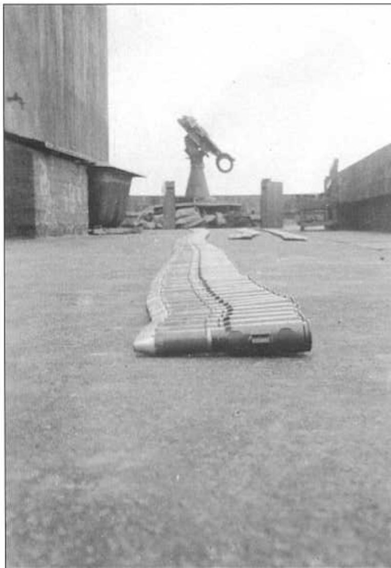
Left: The triplet machine gun MG 151/20 on the lower platform of the Friedrichshain G-Tower with ammunition belts fed from the ammunition boxes in the middle and on both sides, but without a protective shield. The outer belts have 240 rounds each, the inner 500 rounds. Middle: Loaded ammunition belts with 20 mm rounds for the triplet MG 151/20. The shell types were explosive-tracers, with or without fragmentation. Right: The weapon was operated without any range finder and was aimed manually! The gunner simply stood behind the weapon. The three ammunition boxes aren't set up yet.
