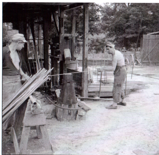
There were severe shortages of raw materials in the Fifties and therefore steel was a valuable commodity. The huge amount of steel reinforcement was salvaged and the bars straightened on special workbenches (see the picture in the middle) and piled up in huge dumps to await transportation.
