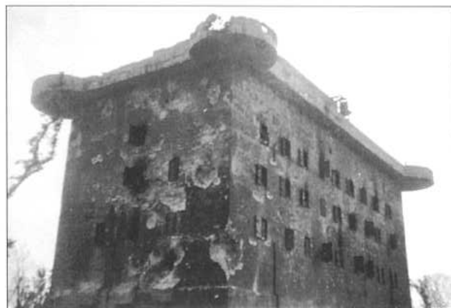
Top: The southern outer wall of the Humboldthain G-Tower shows heavy battle damage. Some sections of the outer walls were riddled with direct hits by artillery shells. Above: the Friedrichshain L-Tower. The Soviet artillery tried to penetrate the outer walls with permanent shelling. Perhaps they succeeded on the front side near the second window under the lower platform. They aimed specifically at the transoms. Left: The last battle has finally come to an end. The heavy Flak has fallen silent. 13 kills were painted on the left barrel.
