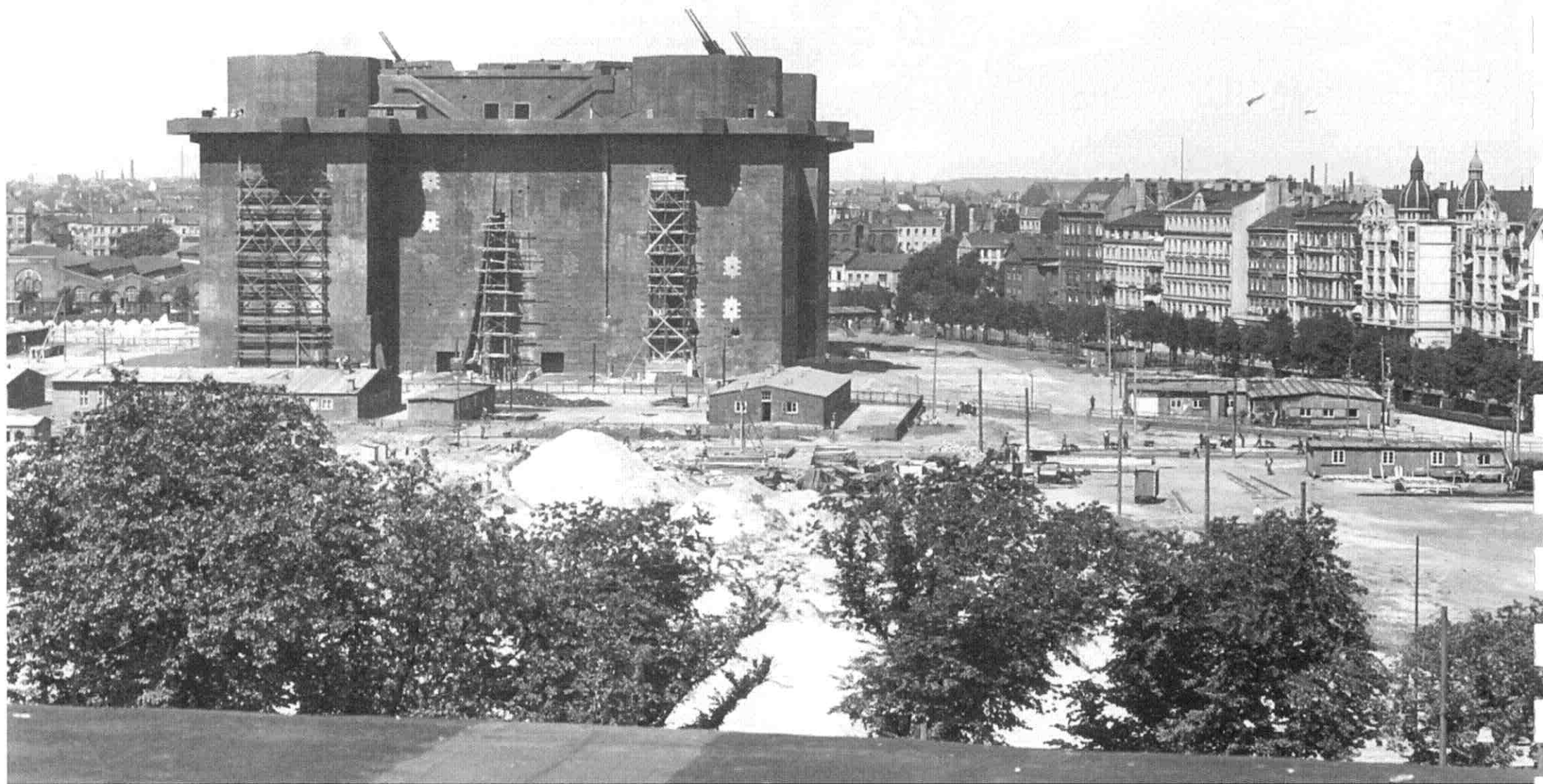
The main body of the Gun Tower at Heiligengeistfeld is complete, parts of the wooden scaffolding can still be seen. All but one of the twin 128 mm AA have already been installed. The white spots on the camouflage paint are interesting, they mark the positions of planned windows. In postwar times, the windows which had only been provisionally bricked up were opened by the OXYGEN Blasting & Building Company. The Gun Tower had a total of 176 windows. The construction site is protected against air attack by several barrage balloons. The external difference compared to the Berlin Gun Towers lies in the design of the projections of the lower platform, which were supported by sturdy beams. The same differences apply to the radar towers.
