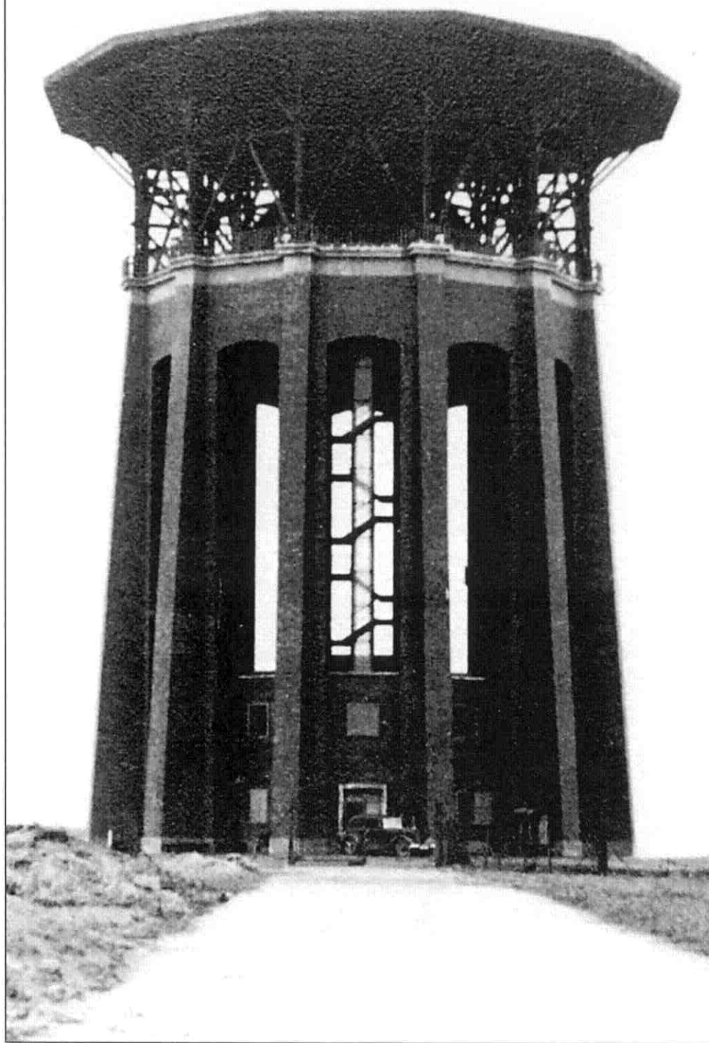
Left: The transmission tower (Project C) was erected in 1941 at a cost of 500,000 RM on a hill near Tremmen in the Havelland area, 40 km west of Berlin. The tower was equipped with the first long range radar (Panoramagerät) with a range of 300 km. The tower was linked by landline to the headquarters of the 1 st AA-Division in the Zoo Flak Tower. When RAF Mosquitos attacked the tower in February 1944, Propaganda Minister Joseph Goebbels wrote resignedly in his diary on 12 th of February 1944, that although the Panoramagerät had survived the raid undamaged, he was depressed to know that the RAF had such intimate knowledge of Berlin's air-defences. Top: Picture from 1942. The long-range radar was a 20 m long beam equipped with 16 dipoles. Bottom: West view of the hill where the transmission tower once stood, blown up after the war by the Russians. Some concrete remains can still be found today.
