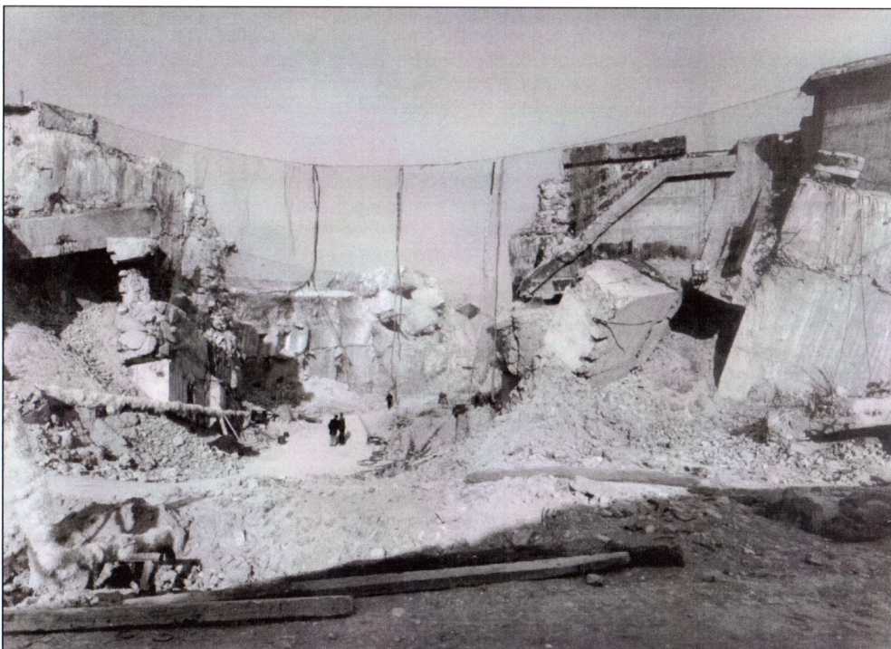
The Zoo G-Tower had to be cleared of ammunition before blasting could take place. Soviet artillery shells were lodged in the outer walls (top left) and some slabs of British explosives which had failed to detonate during earlier blasting attempts were found inside the Flak tower (top). In total 800 blastings were carried out (top right). To avoid damage caused by flying concrete fragments and other debris, huge torpedo-nets were brought from Hamburg and stretched over the building's area (bottom). For a while, the Technical Support Organisation (THW) in Berlin used thermal lances to cut the concrete walls (bottom right).
