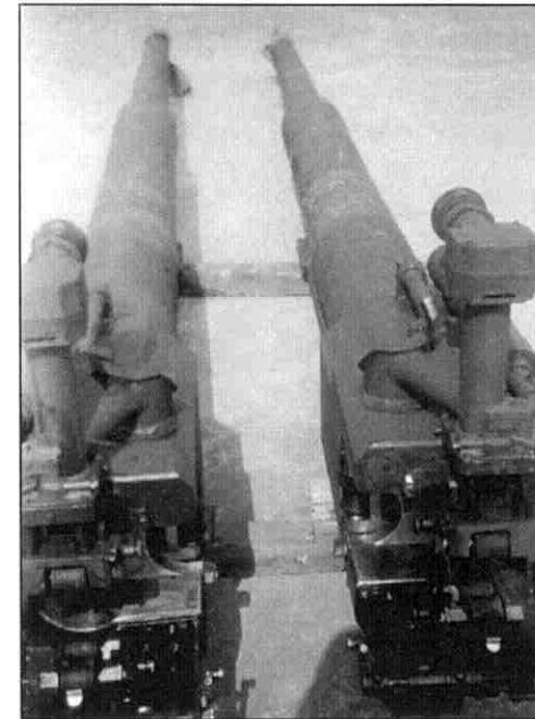
Both the tower crane as well as external cranes were used to lift the heavy 27 tonne AA-guns onto the top of the G-Tower. The guns had to be disassembled first. Top left: Each barrel was transported individually onto the top of the Friedrichshain G-Tower and stored there for a while (top right). Then the first AA-guns were assembled and mounted on their plinths.
