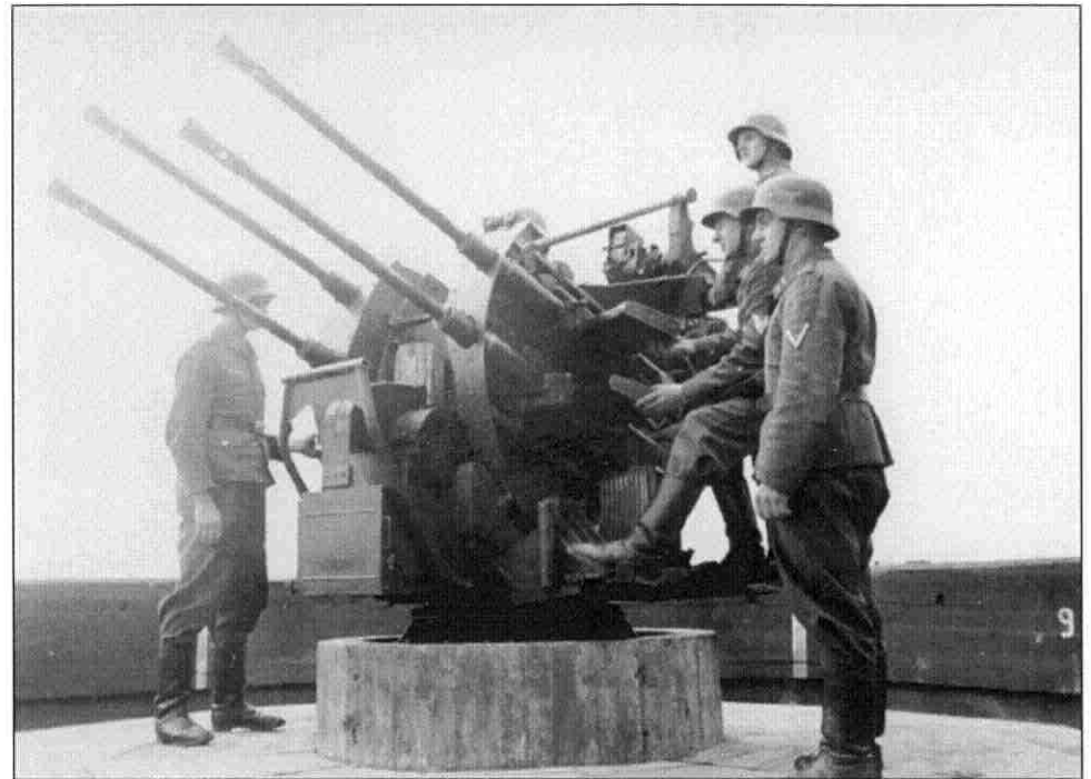
The L-Towers and the lower platforms of the G-Towers were equipped with light AA guns to combat fighter planes. The most effective weapon was the 20 mm four-barrelled Mk 38 gun, originally mounted on wooden pedestals, which would later be replaced due to the fire risk. Top right: A concrete plinth with a 20 mm quad mounted on the Heiligengeistfeld G-Tower, Hamburg. Markings were painted on the inside of the balustrade to help with direction finding and calculating range. The wavy lines painted (bottom left) on Flak towers in Berlin were intended as tracking indicators for the light AA. Bottom: Luftwaffenhelfer in fatigues: gun crews of the 20 mm Mk 38 quads mounted on the Friedrichshain L and G-Towers (left and right).
