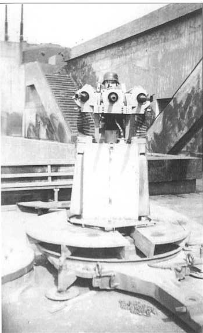
Left: The triplet machine gun MG 151/20 on the lower platform of the Friedrichshain G-Tower with ammunition belts fed from the ammunition boxes in the middle and on both sides, but without a protective shield. The outer belts have 240 rounds each, the inner 500 rounds. Middle: Loaded ammunition belts with 20 mm rounds for the triplet MG 151/20. The shell types were explosive-tracers, with or without fragmentation. Right: The weapon was operated without any range finder and was aimed manually! The gunner simply stood behind the weapon. The three ammunition boxes aren't set up yet.
