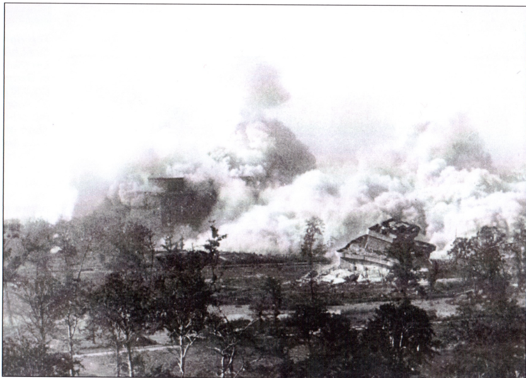
British ground floor plan of the Zoo Gun-Tower shows the distribution of the ammunition. Top right: In August 1947 British insert charges into the bore-holes. Right: On July 30 th 1948 the G-Tower was blown up with 35 tonnes of explosives and finally destroyed after several attempts had failed.
