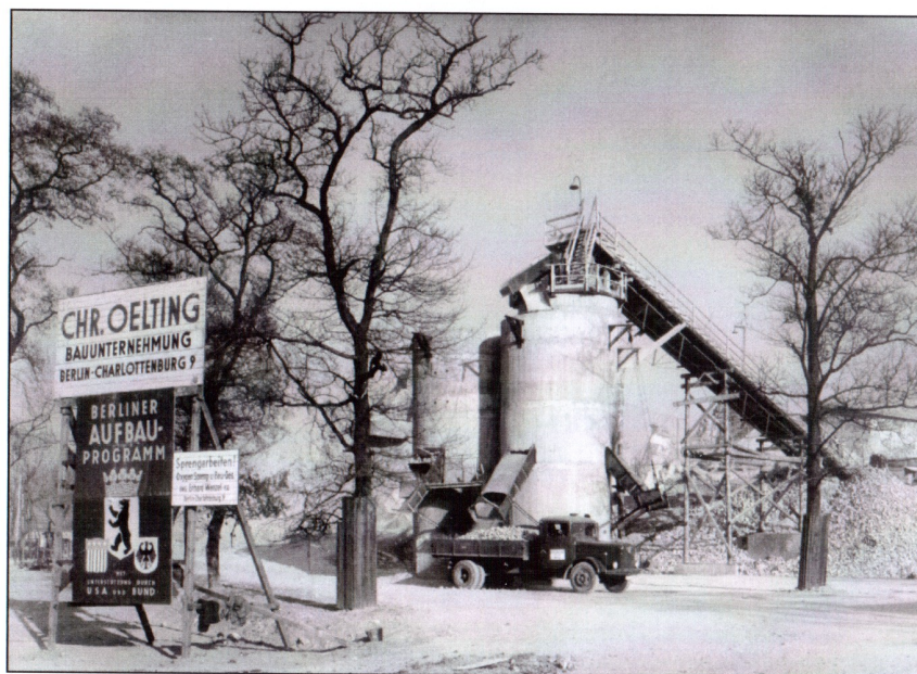
Left. The concrete was recycled too. The Oelting Company from Pinneberg built concrete silos for the recovered gravel, and the ground-up building materials of the former Flak tower was loaded from the silos onto trucks via chutes. The ground concrete was used for the underground railway as well as for road building. Right: The destruction of the Zoo Flak tower is nearly complete on March 15 th 1958. Only the massive foundation with some 17,600 m 3 of reinforced concrete still lay in the ground until it was finally removed in 1969-70.
