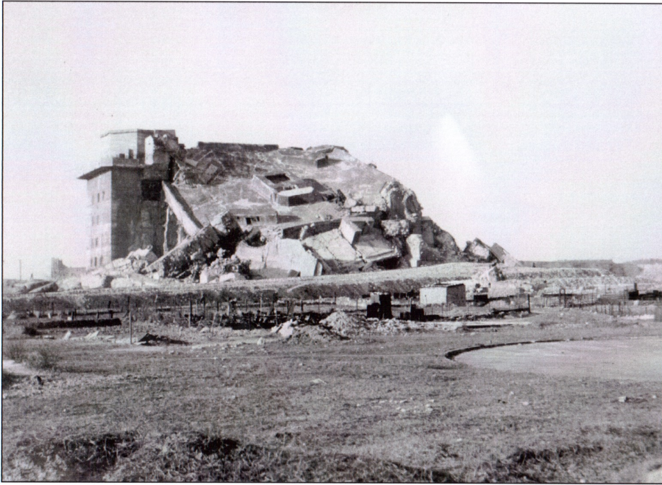
Top: Both southern towers and the outer wall between them collapsed after the third blasting on March 13 th 1948, using 25 tonnes of explosives. Right: Relief workers are covering the Humboldt G-Tower with the debris of 4,000 dwellings or 1.6 million cubic meters of rubble. In 1950 some 1,300 relief workers were employed on the "Rubble Mountain" site. Bottom left: The L-Tower after the blast on December 13 th 1947 which used 16 tonnes of explosives. The upper row of windows and the wall fragment can still be seen today. The bunker has disappeared under earth and rubble up to this height. In the background on the right is the G-tower. Bottom right: The L-tower on Gustav-Meyer-Allee after being buried.
