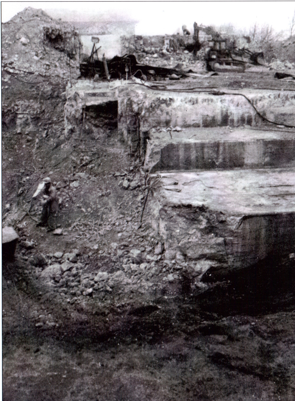
Left: Additional discussions concerning the removal of the 3.2 m thick foundation plate with its 6,152 cubic metres had calculated 55 working days. The problem of how to remove the foundations by blasting but without damaging the sewers below was solved. Photo taken on January 20 th 1975. On the right: After the demolition and removal of the foundations, there was a nine-meter deep excavation, which had to be filled in by the Oxygen company. Bottom right: The Deutsche Telekom building which replaced the Heiligengeistfeld L-
