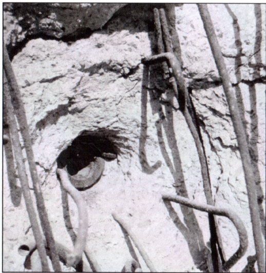
The Zoo G-Tower had to be cleared of ammunition before blasting could take place. Soviet artillery shells were lodged in the outer walls (top left) and some slabs of British explosives which had failed to detonate during earlier blasting attempts were found inside the Flak tower (top). In total 800 blastings were carried out (top right). To avoid damage caused by flying concrete fragments and other debris, huge torpedo-nets were brought from Hamburg and stretched over the building's area (bottom). For a while, the Technical Support Organisation (THW) in Berlin used thermal lances to cut the concrete walls (bottom right).
