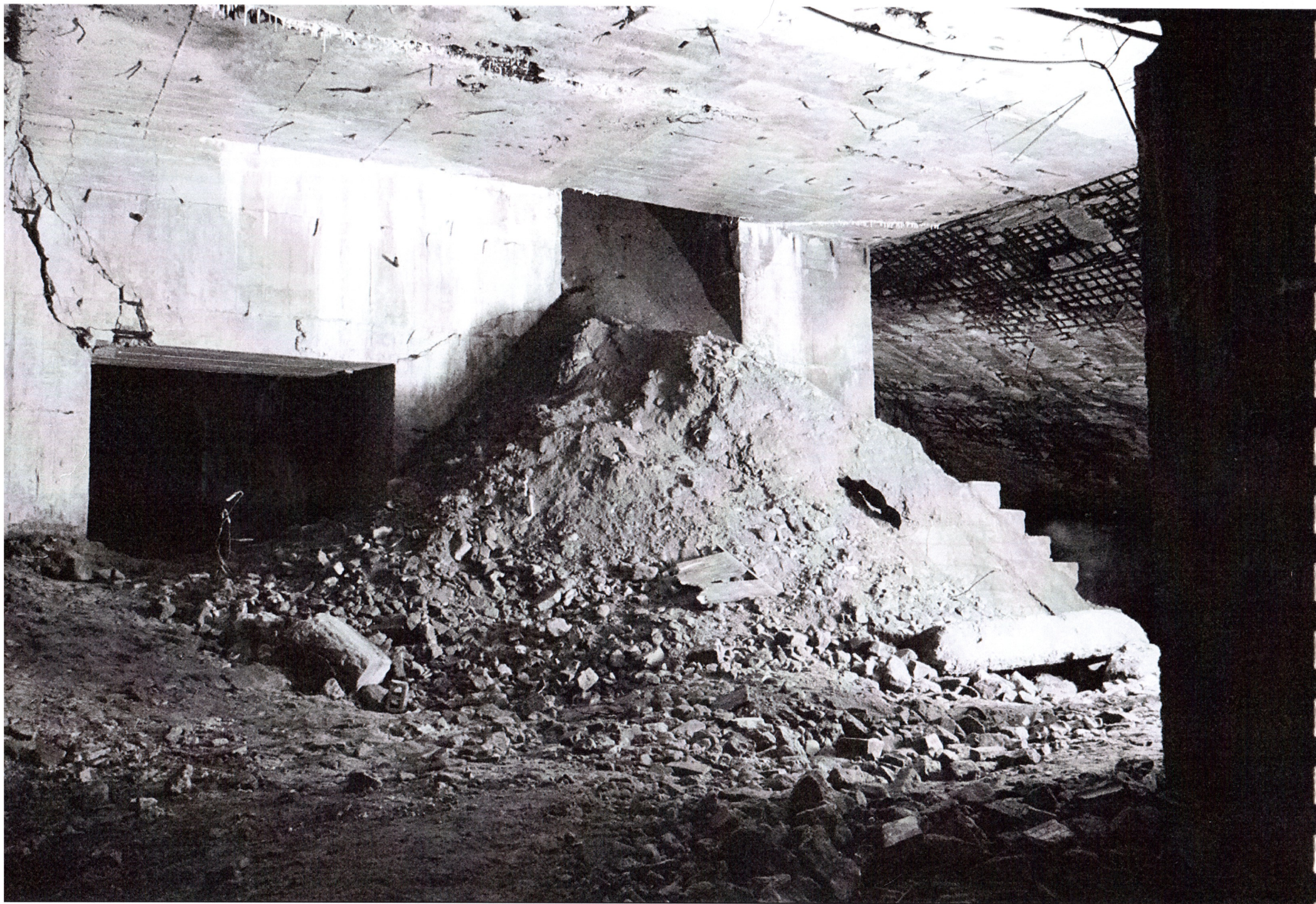
Mounds of debris and rubble in the Humboldtsein G-Tower. The ceiling is crushed on the right side after the blasting carried out by French engineers in March 1949, when the
