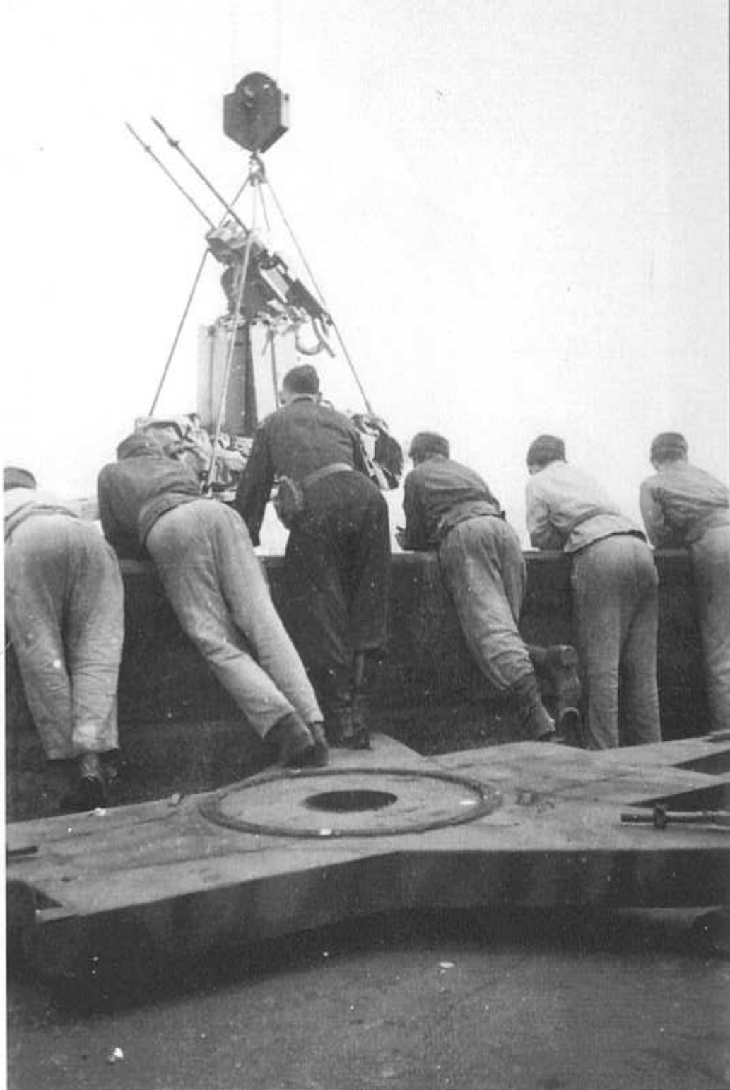
Left: While the fixed cross carriage 151/7 has already been hoisted onto the lower platform, the triplet machine gun (the centre barrel has been temporary removed) is being installed by a crane. Top: Setting up the triplet machine gun 151/20 on its pedestal and carriage. Around the plinth are the ammunition boxes, containing the ammunition belts to feed the three-barrelled gun. The weight of the MG 151/20 (barrel and breech) was 42 kg, the muzzle velocity 790 m/sec. elevation -10^{\circ} to +60^{\circ} . Bottom: Two MG 151/20s with missing middle barrels. Bottom left one can see 128 mm barrels.
