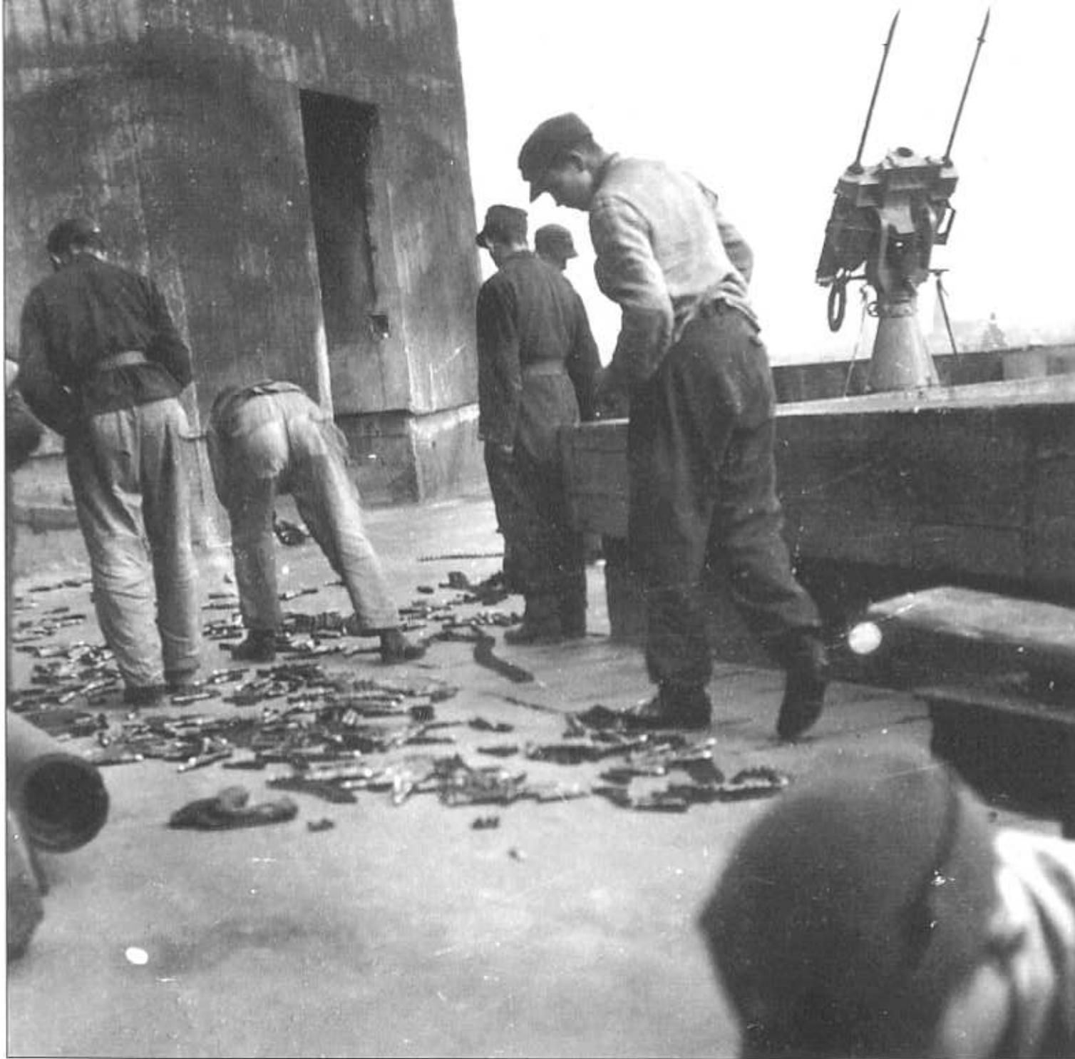
Left: On the ground of the lower platform of the Friedrichshain G-Tower are many 20 mm cartridges for the triplet machine gun MG 151/20 (in the background). The barrel in the middle is temporary removed. Clearly visible are the outer slanted blast pipes to reduce the torque caused by the recoil of the outer barrels. Without the ammunition cases, the bracket is visible. On the bottom left is the rounded shoulder support.
