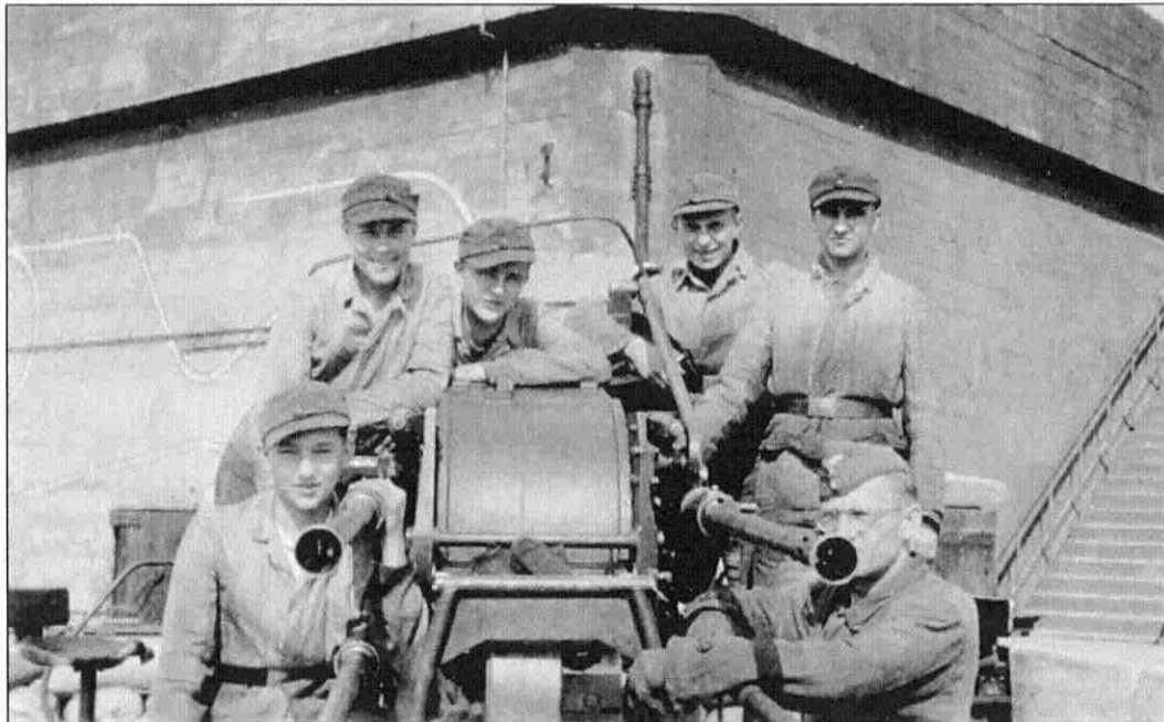
The L-Towers and the lower platforms of the G-Towers were equipped with light AA guns to combat fighter planes. The most effective weapon was the 20 mm four-barrelled Mk 38 gun, originally mounted on wooden pedestals, which would later be replaced due to the fire risk. Top right: A concrete plinth with a 20 mm quad mounted on the Heiligengeistfeld G-Tower, Hamburg. Markings were painted on the inside of the balustrade to help with direction finding and calculating range. The wavy lines painted (bottom left) on Flak towers in Berlin were intended as tracking indicators for the light AA. Bottom: Luftwaffenhelfer in fatigues: gun crews of the 20 mm Mk 38 quads mounted on the Friedrichshain L and G-Towers (left and right).
