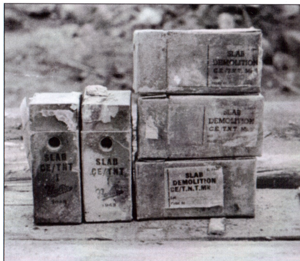
The Zoo G-Tower had to be cleared of ammunition before blasting could take place. Soviet artillery shells were lodged in the outer walls (top left) and some slabs of British explosives which had failed to detonate during earlier blasting attempts were found inside the Flak tower (top). In total 800 blastings were carried out (top right). To avoid damage caused by flying concrete fragments and other debris, huge torpedo-nets were brought from Hamburg and stretched over the building's area (bottom). For a while, the Technical Support Organisation (THW) in Berlin used thermal lances to cut the concrete walls (bottom right).
