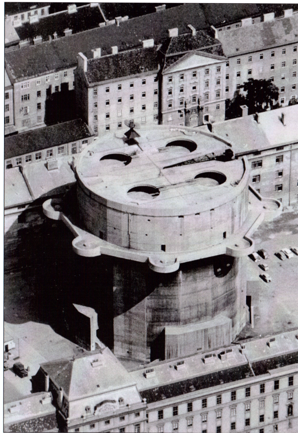
Top: This picture was taken in 1995 from a nearby multi-storey car park. The first platform shows the lobes with splinter-proof entrances. The camouflage paint on the top of the tower is completely gone. Since the Austrian Armed Forces were running this bunker, some radar dishes were fitted to the reinforced concrete wall. Right: Several years later: rain and snow have already washed the camouflage paint away. On the top of the G-Tower, the recesses for the 128 mm Flak and for the crane, when not in operational position. The three entrances are protected by bombproof constructions, built in 1944. Bottom: After the war the Stiftskaserne G-Tower became a US ordnance base. The G-Tower is still painted with camouflage colours, only the lower part was painted white to make orientation easier during the Blackout.
