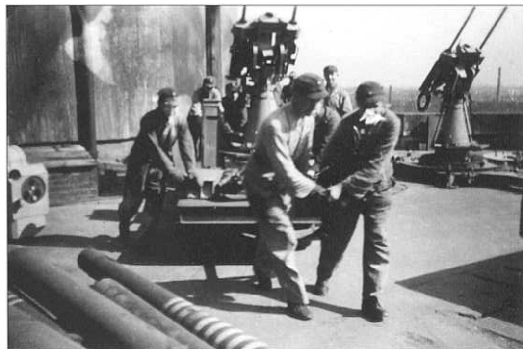
Left: While the fixed cross carriage 151/7 has already been hoisted onto the lower platform, the triplet machine gun (the centre barrel has been temporary removed) is being installed by a crane. Top: Setting up the triplet machine gun 151/20 on its pedestal and carriage. Around the plinth are the ammunition boxes, containing the ammunition belts to feed the three-barrelled gun. The weight of the MG 151/20 (barrel and breech) was 42 kg, the muzzle velocity 790 m/sec. elevation -10^{\circ} to +60^{\circ} . Bottom: Two MG 151/20s with missing middle barrels. Bottom left one can see 128 mm barrels.
