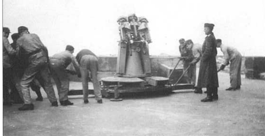
Left: While the fixed cross carriage 151/7 has already been hoisted onto the lower platform, the triplet machine gun (the centre barrel has been temporary removed) is being installed by a crane. Top: Setting up the triplet machine gun 151/20 on its pedestal and carriage. Around the plinth are the ammunition boxes, containing the ammunition belts to feed the three-barrelled gun. The weight of the MG 151/20 (barrel and breech) was 42 kg, the muzzle velocity 790 m/sec. elevation -10^{\circ} to +60^{\circ} . Bottom: Two MG 151/20s with missing middle barrels. Bottom left one can see 128 mm barrels.
