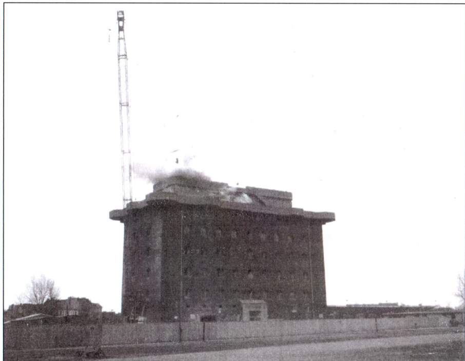
Top left: Probably one of the first blastings in December 1973 was to make an entrance for the tracked vehicle. The fifth floor with its staircases leading to the interior seems to be undamaged.
