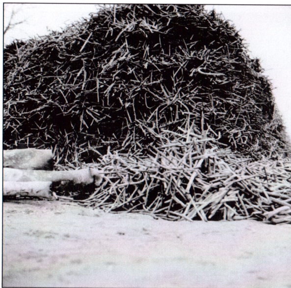
There were severe shortages of raw materials in the Fifties and therefore steel was a valuable commodity. The huge amount of steel reinforcement was salvaged and the bars straightened on special workbenches (see the picture in the middle) and piled up in huge dumps to await transportation.
