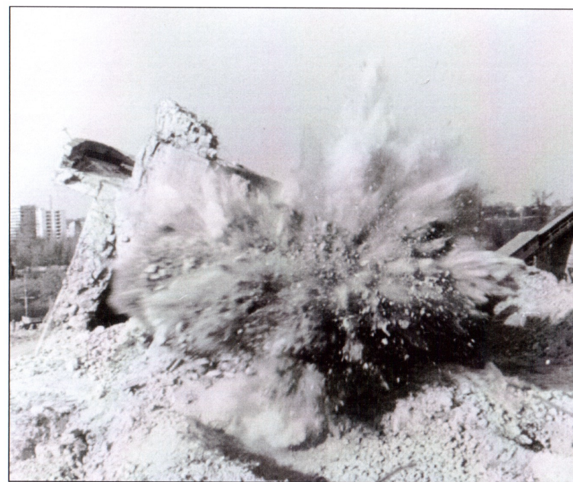
The Zoo G-Tower had to be cleared of ammunition before blasting could take place. Soviet artillery shells were lodged in the outer walls (top left) and some slabs of British explosives which had failed to detonate during earlier blasting attempts were found inside the Flak tower (top). In total 800 blastings were carried out (top right). To avoid damage caused by flying concrete fragments and other debris, huge torpedo-nets were brought from Hamburg and stretched over the building's area (bottom). For a while, the Technical Support Organisation (THW) in Berlin used thermal lances to cut the concrete walls (bottom right).
