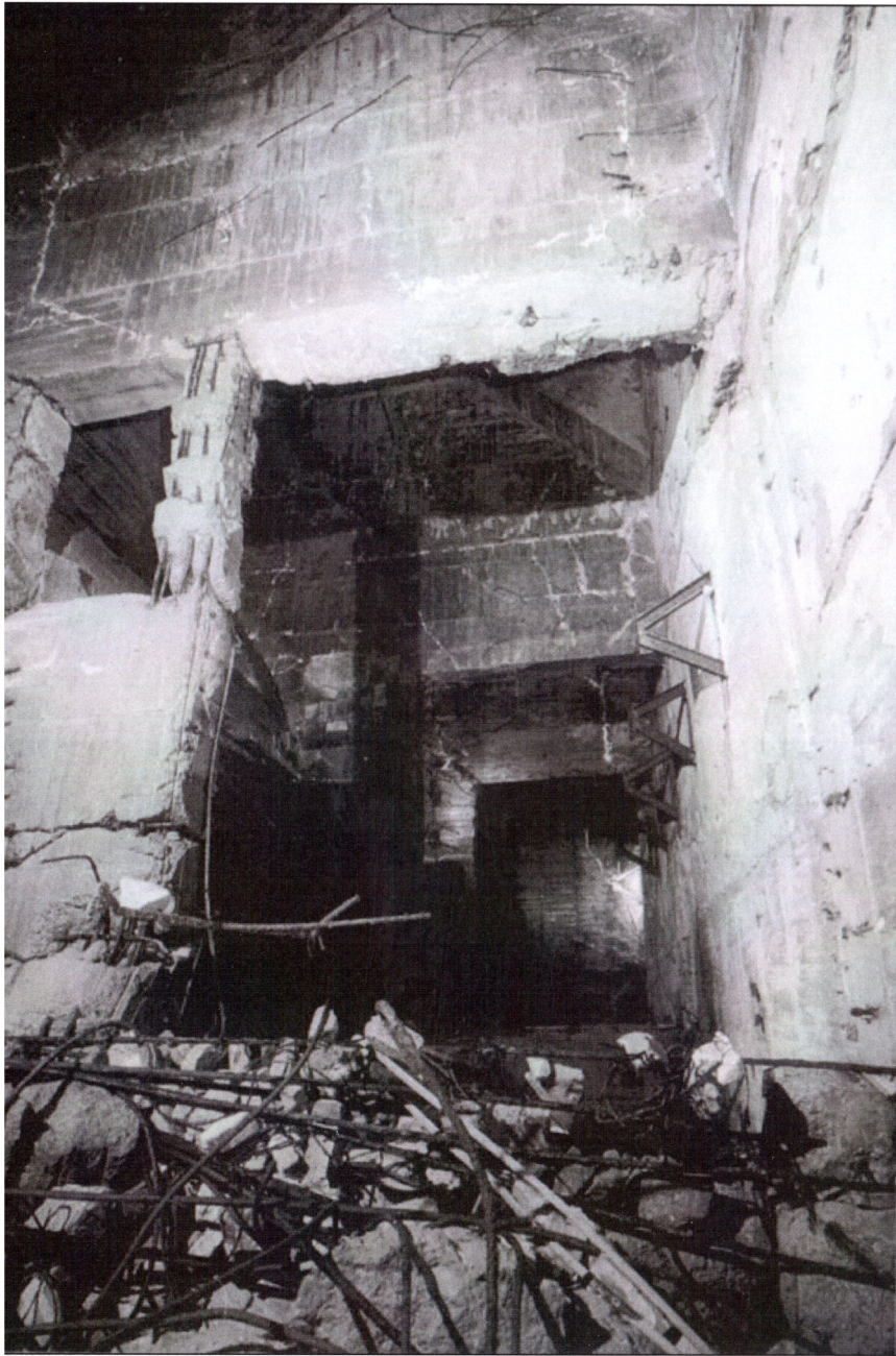
Left top: Surveying in the area of tower 3, on the left hand side the spiral staircase, on the right the shaft for the goods lift. Right: View into the 20 m p spiral staircase, which steps were destroyed during the blast in March, 8. Top: Shaft of the goods lift, becoming a paradise for rats, when soviet liers in 1945 dumped all the food stored in the Flak – Tower.
